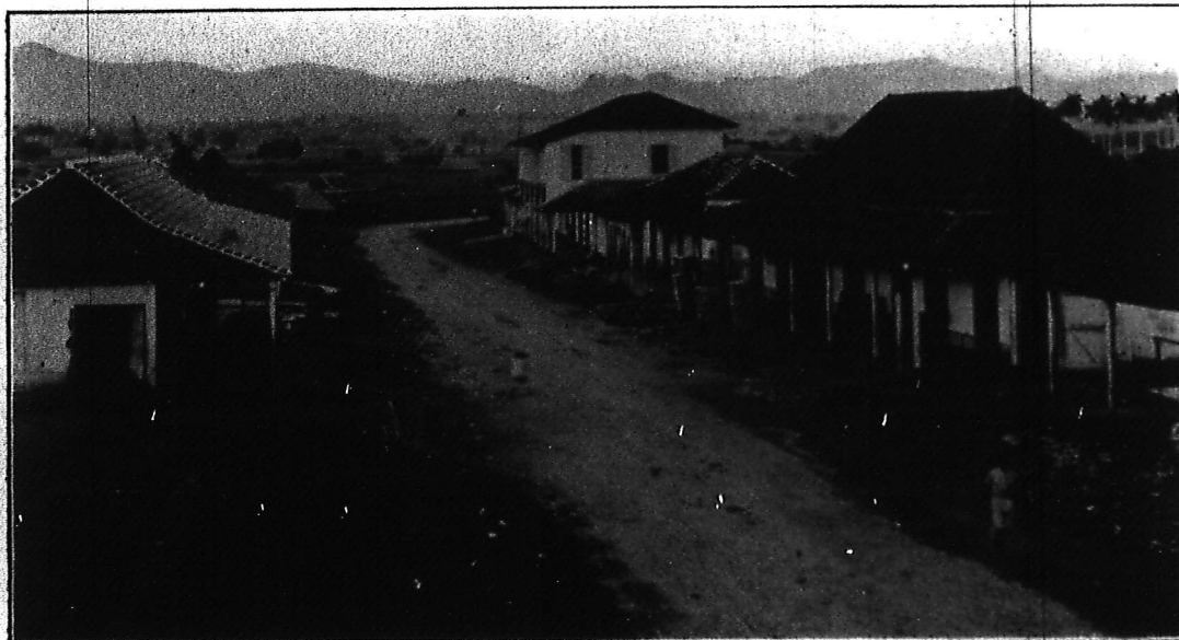
CUBAN VILLAGE WITH BAD TURN ON ROAD
