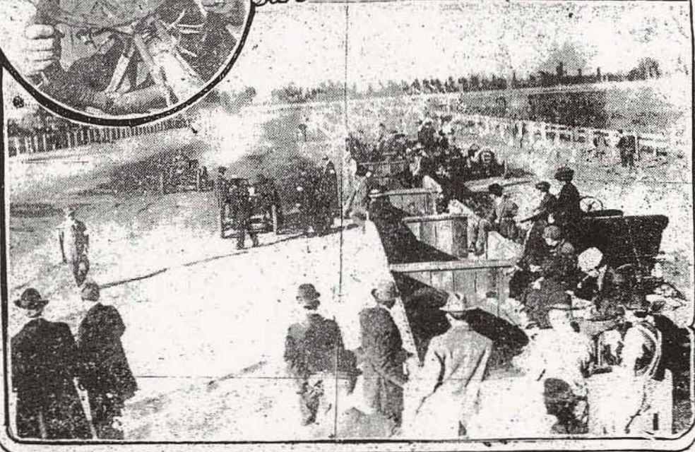
In the repair pits.
