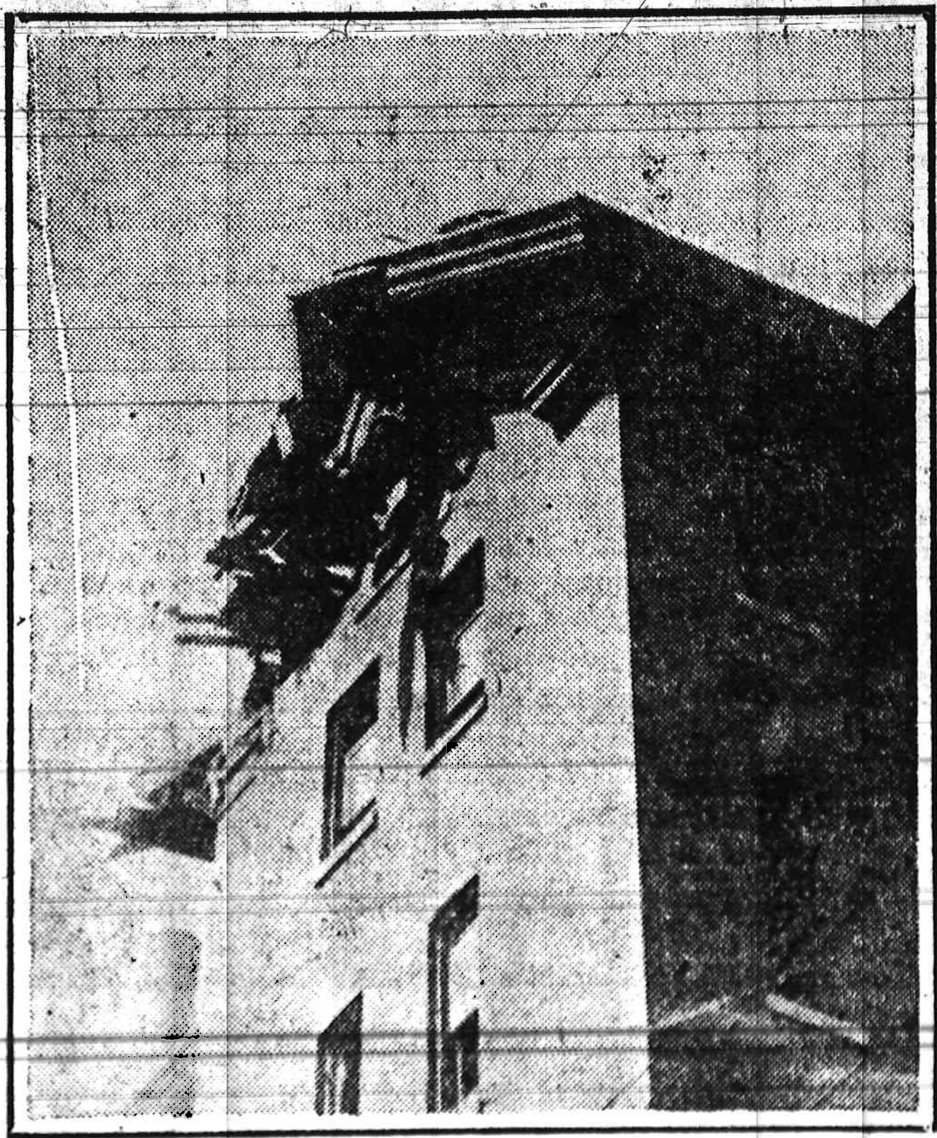
The Prest-o-Lite explosion carried a way a portion of an east gable of St. Vincent's Hospital.
