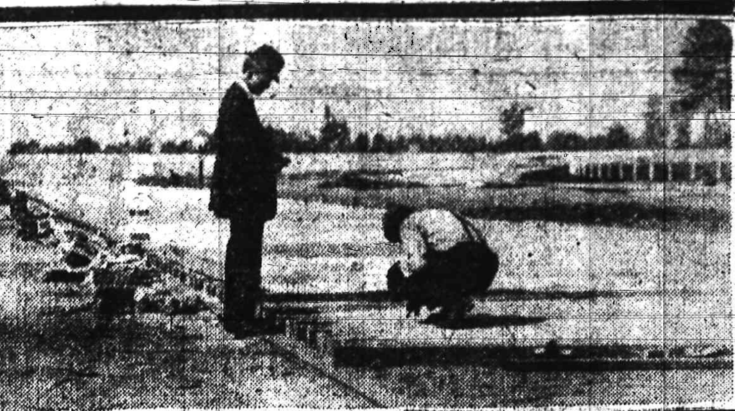
LAYING NEW BRICK ROADWAY
